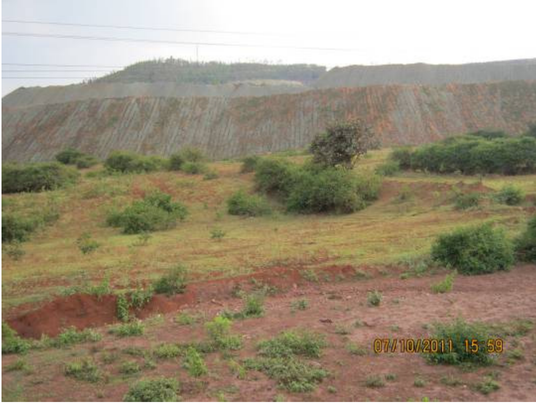
Geo-textile stabilization of steep slopes of OB dumps of Sea Goa mines of Chitradurga
