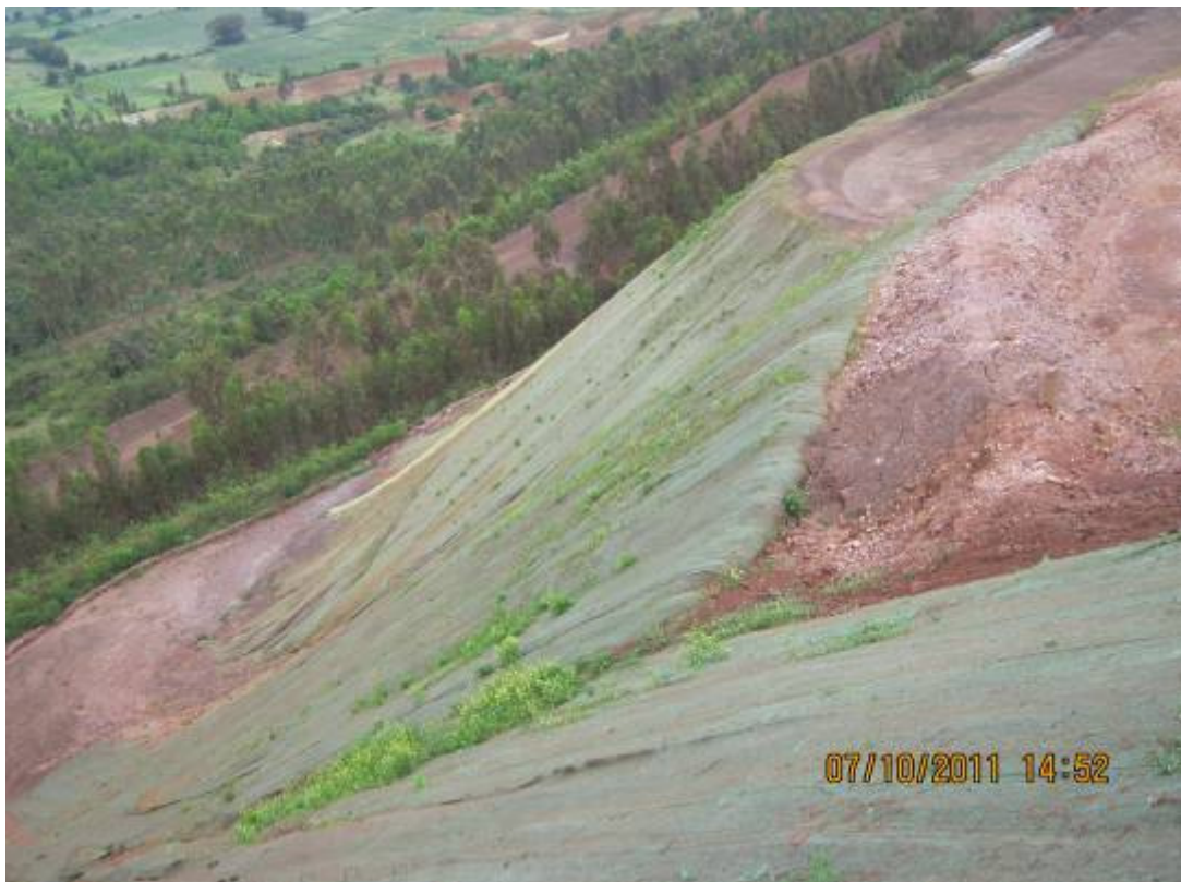
Geo-textile stabilization of steep slopes of OB dump of John mines of Chitradurga
