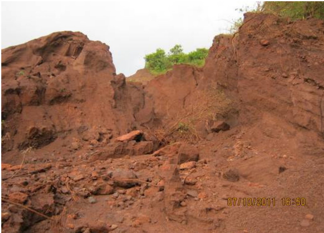
Breaching of OB dump of MEL mines towards forest in Chitradurga
