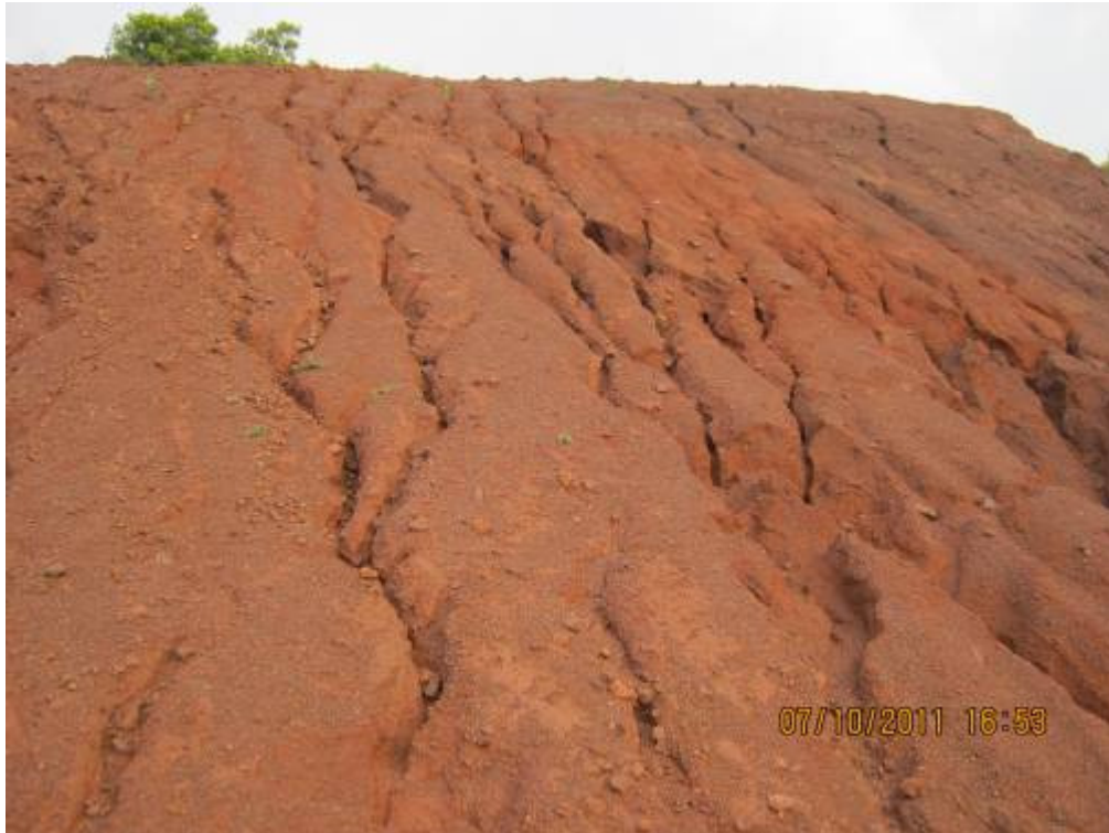
Unstabilized dump of MEL mines of Chitradurga
