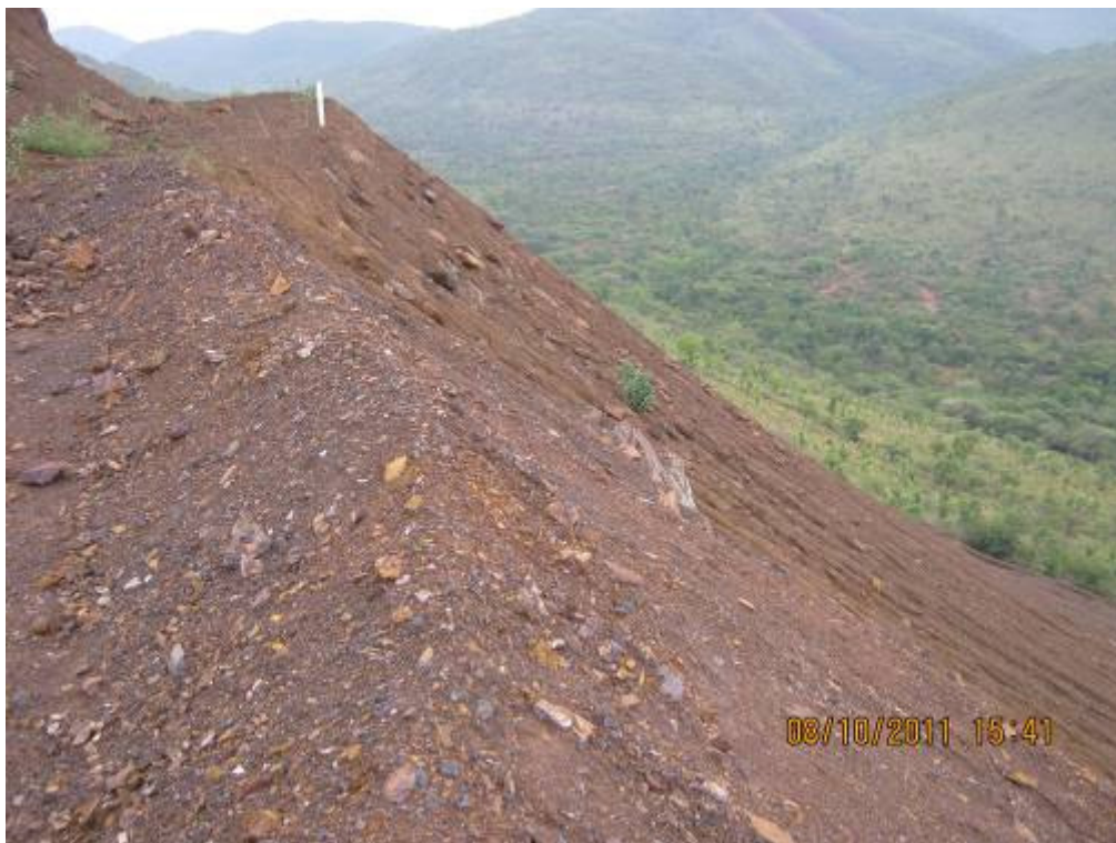
Unstabilized steep OB dump sliding towards vegetation of Allum Veerabhadrapa mines, Chitradurga
