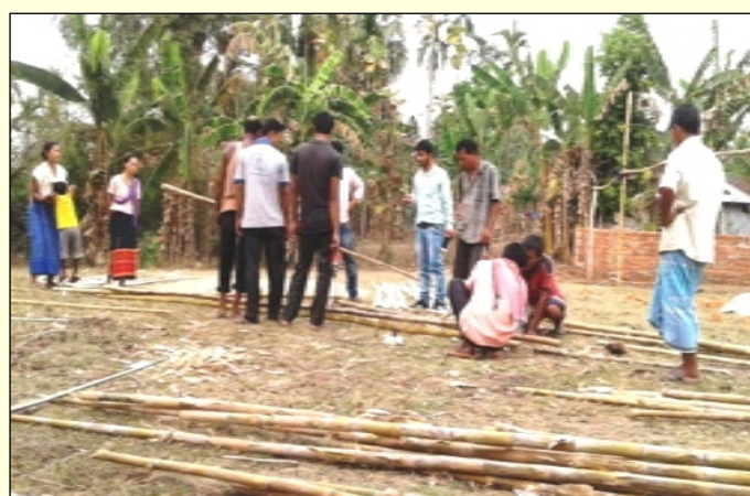
Training on Bamboo preservation, joints and joinery Techniques & tress making
